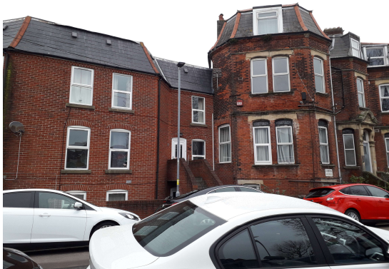
Application site: modern extension connecting to original building
